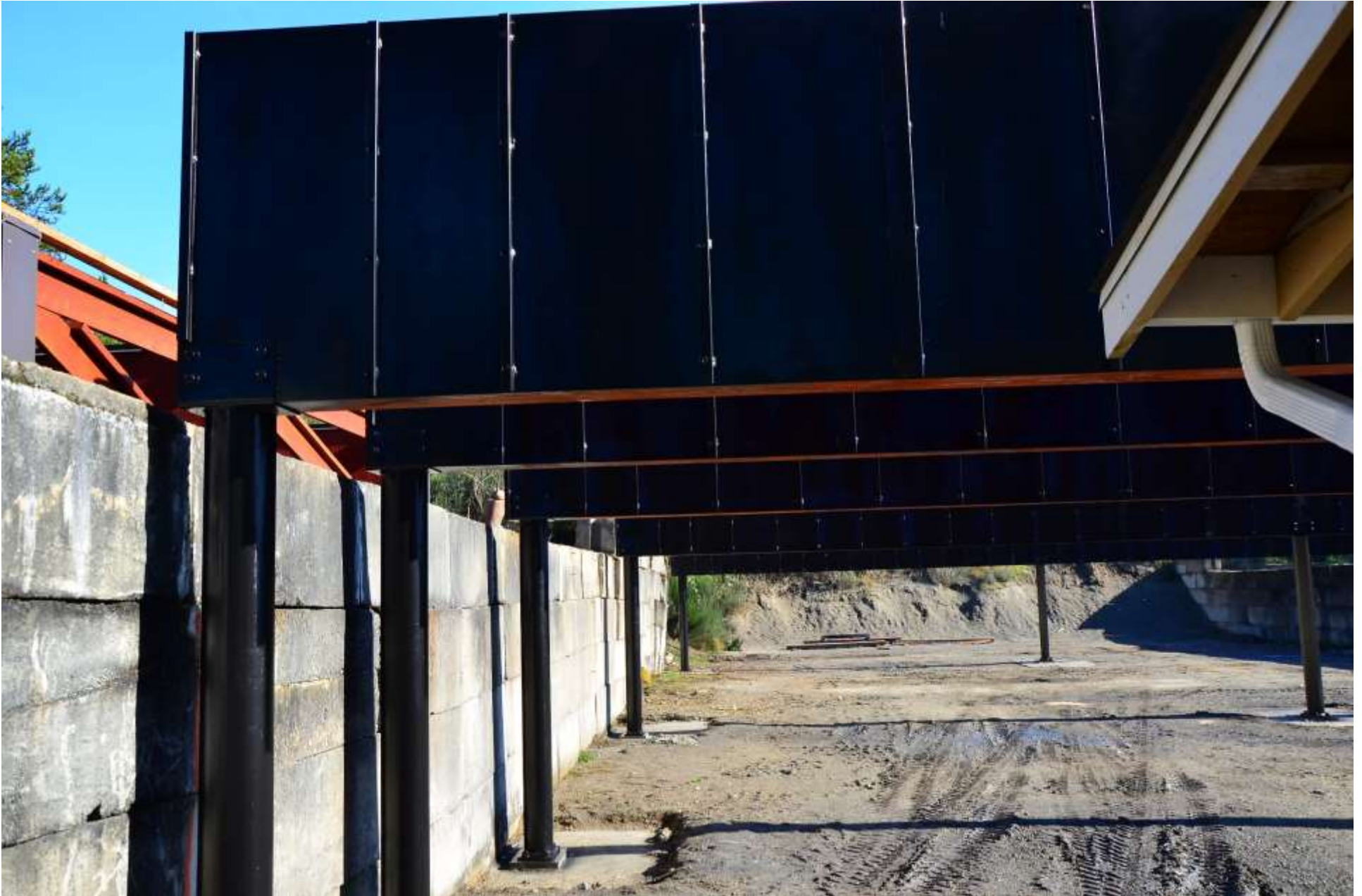
View toward the impact berm.
