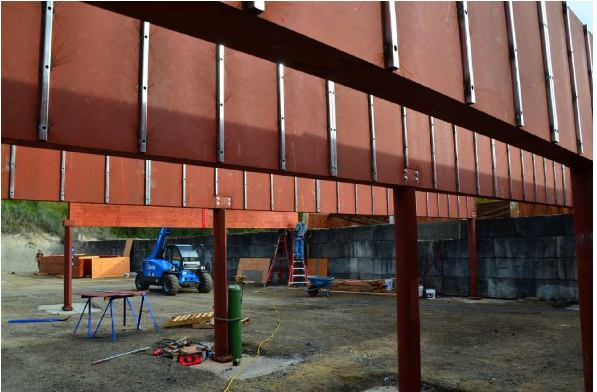
New beam being set into place.
