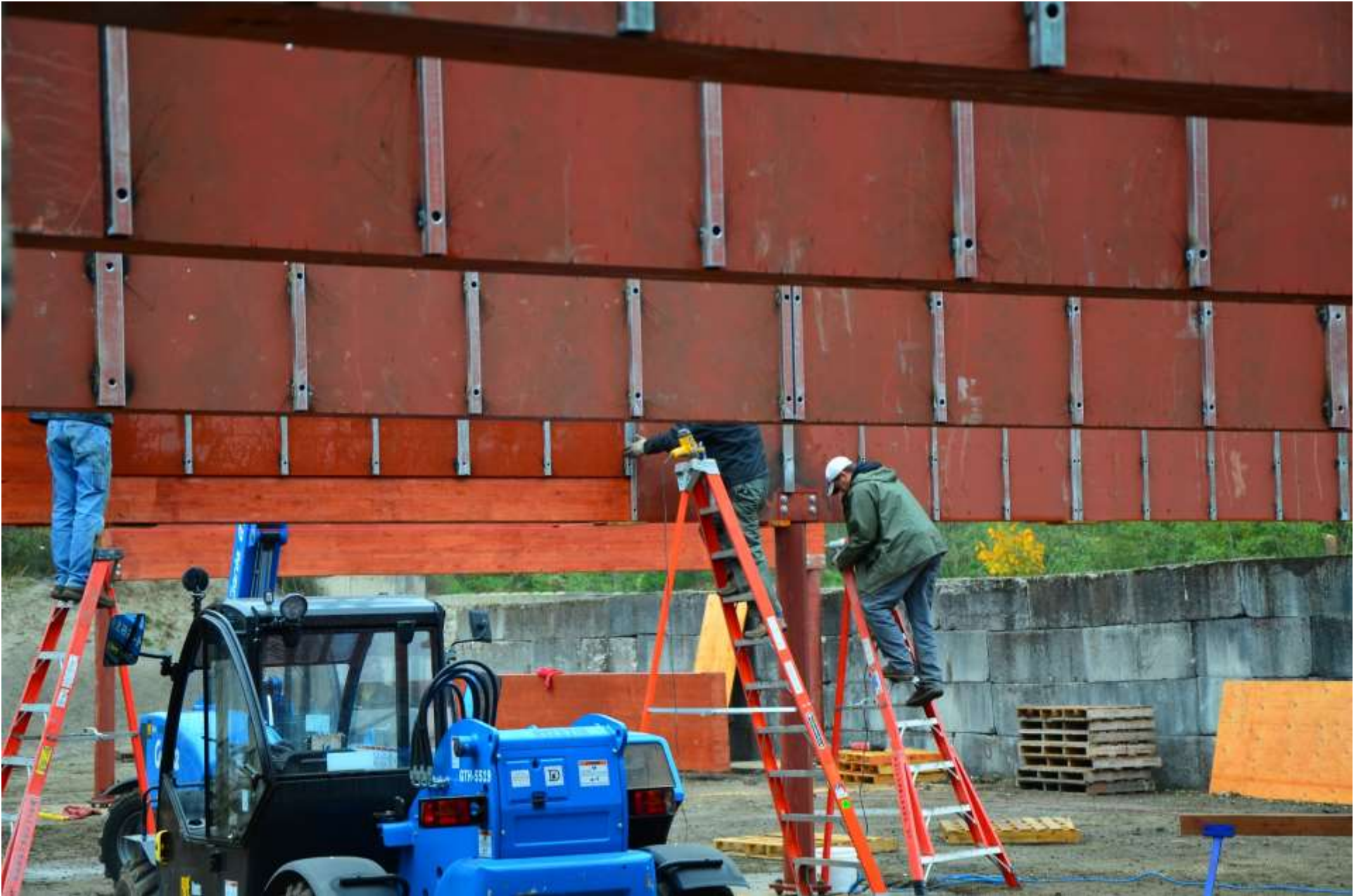
Steel plates being positioned.
