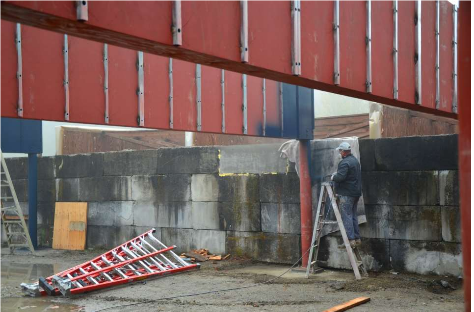
First coats of paint.
