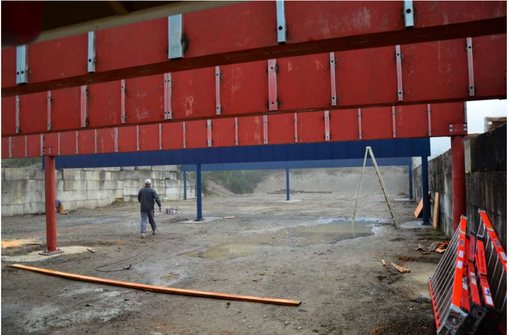
First coats of paint.
