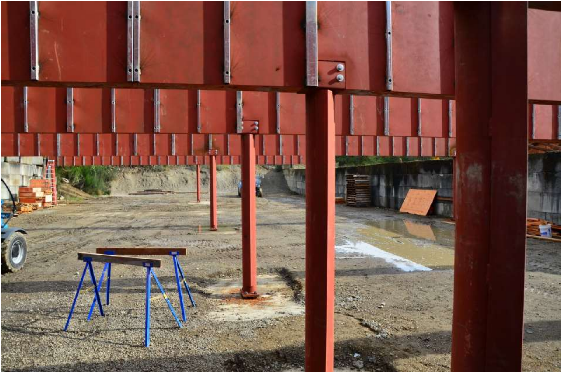
All beams and steel plates in place.
