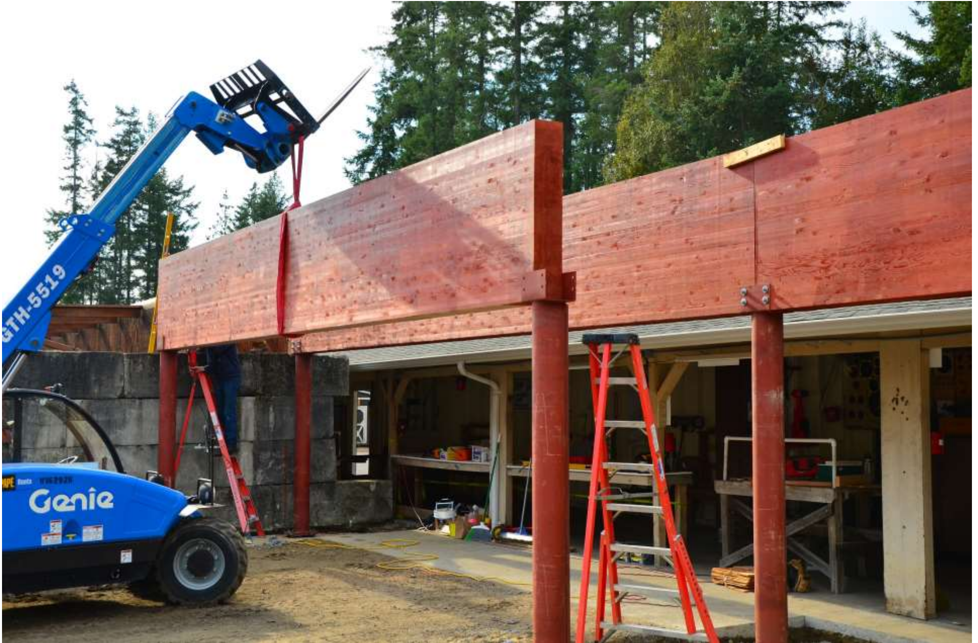
New beam being set into place.
