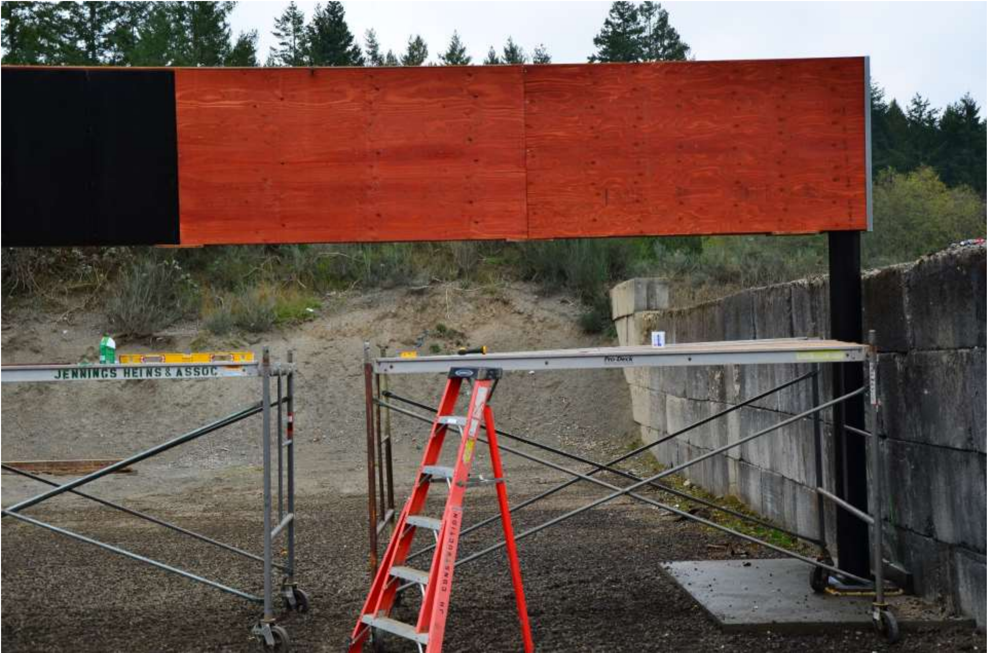
The first of the plywood.
