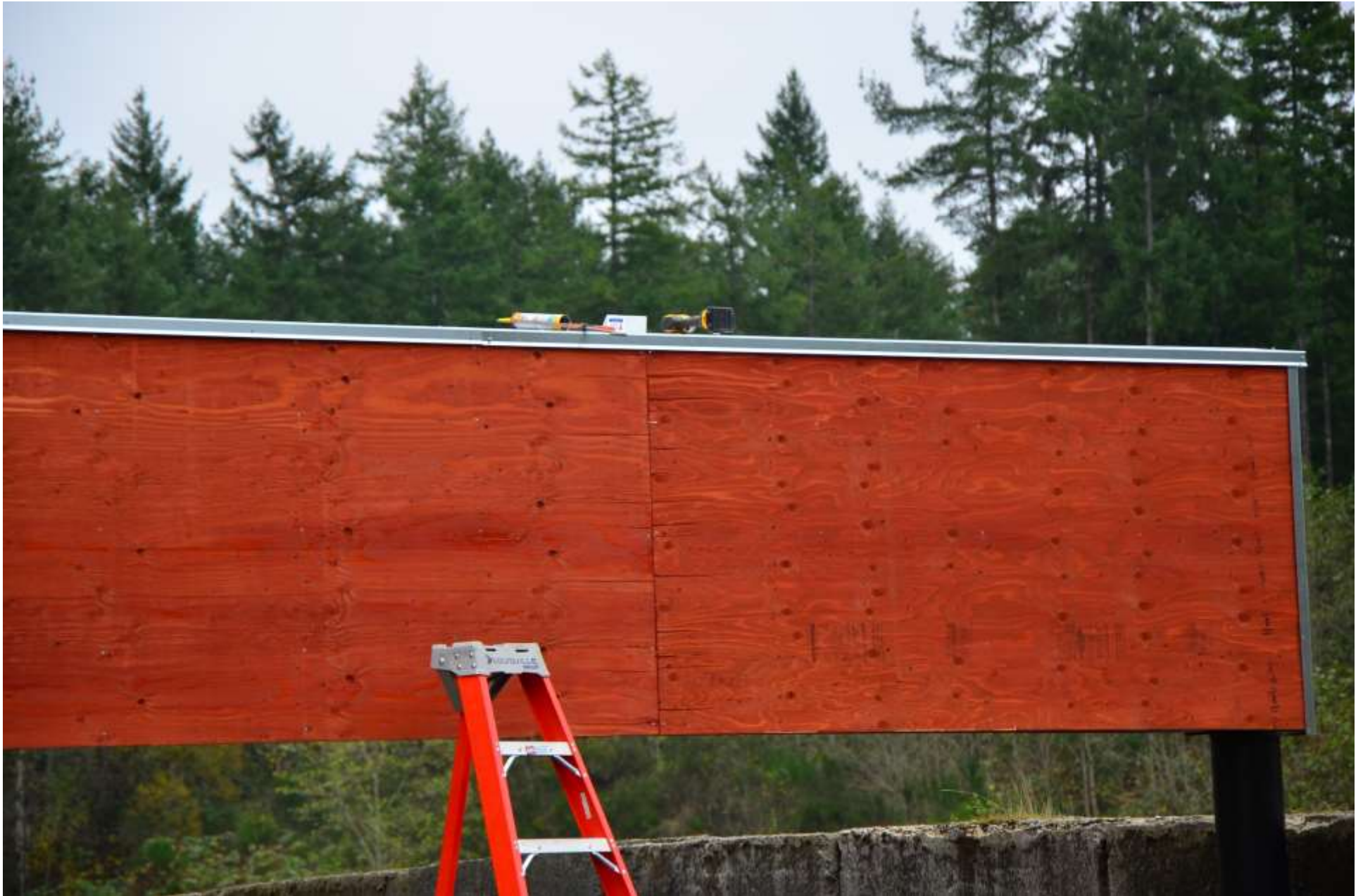
Closer view of the flashing.
