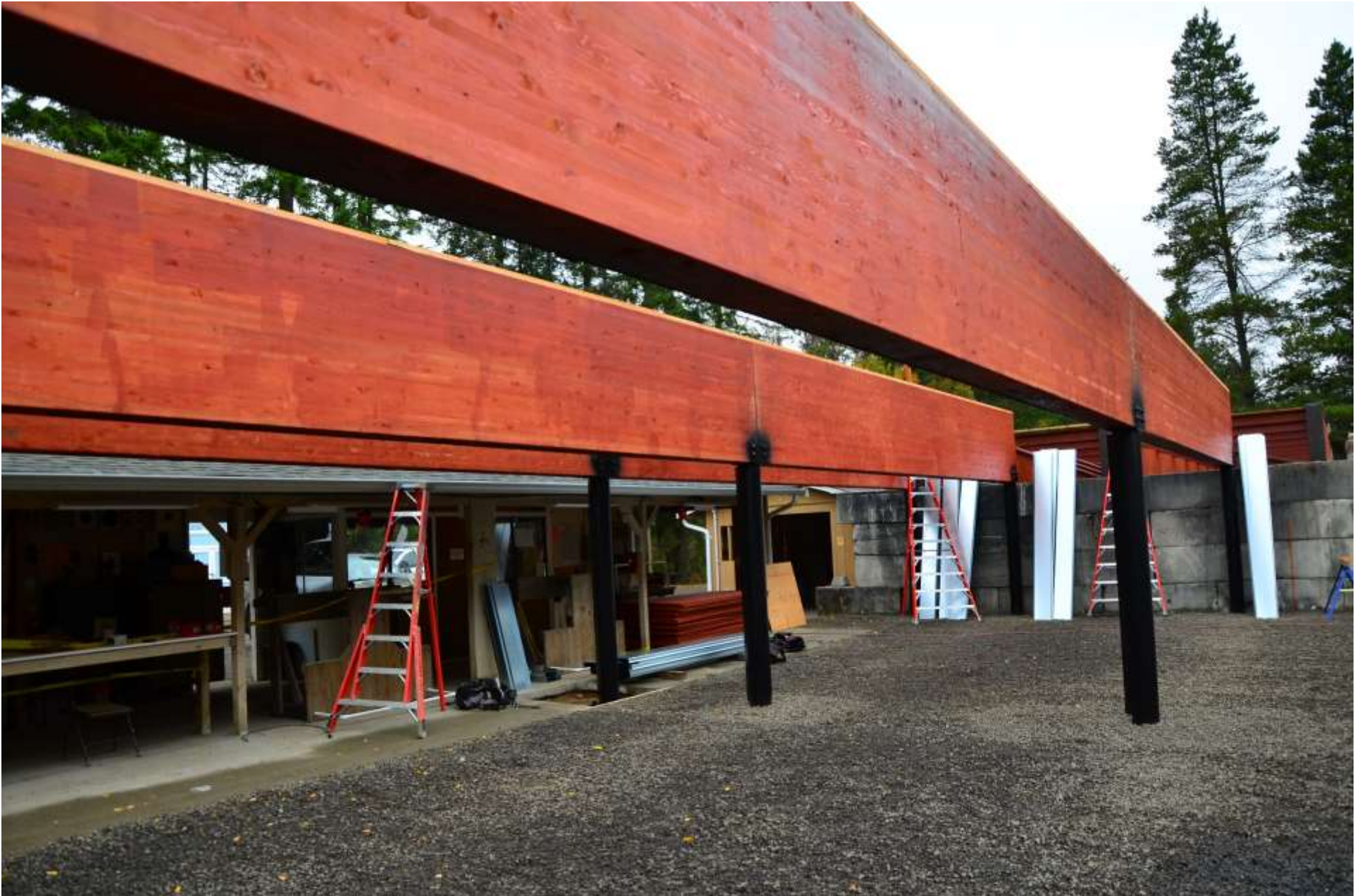
Flashing and top cap view from the back side.
