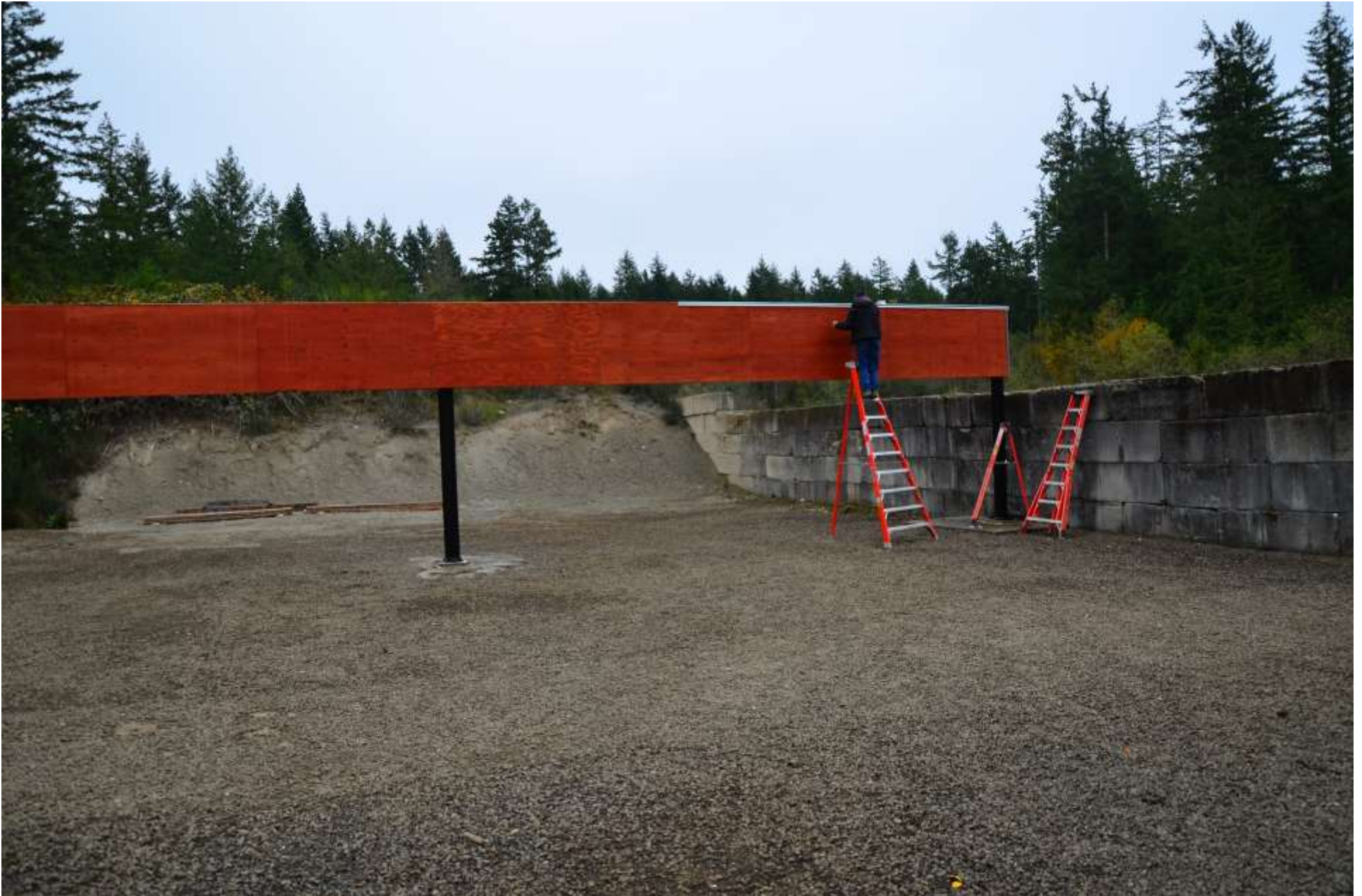
First of the flashing.
